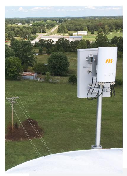
The water tower at Eldridge was an ideal location to deploy wireless Internet radios and antennas to reach the community with reliable Internet service.
