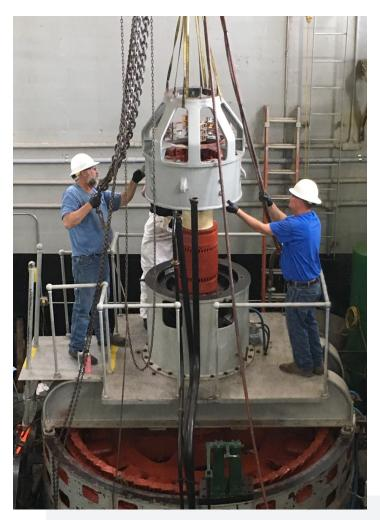
Substation Foreman Richard Newell and Substation Mechanic Chris Miller lower the rebuilt exciter onto the generator shaft of unit #2 at Tunnel Dam Hydo Generating facility.
